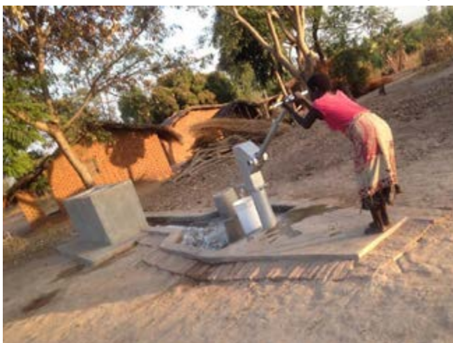
Bohrloch in Gangala
